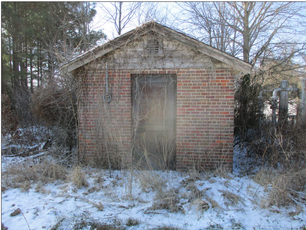
Figure 10. Eastern end of project route at compressor station, view south.
