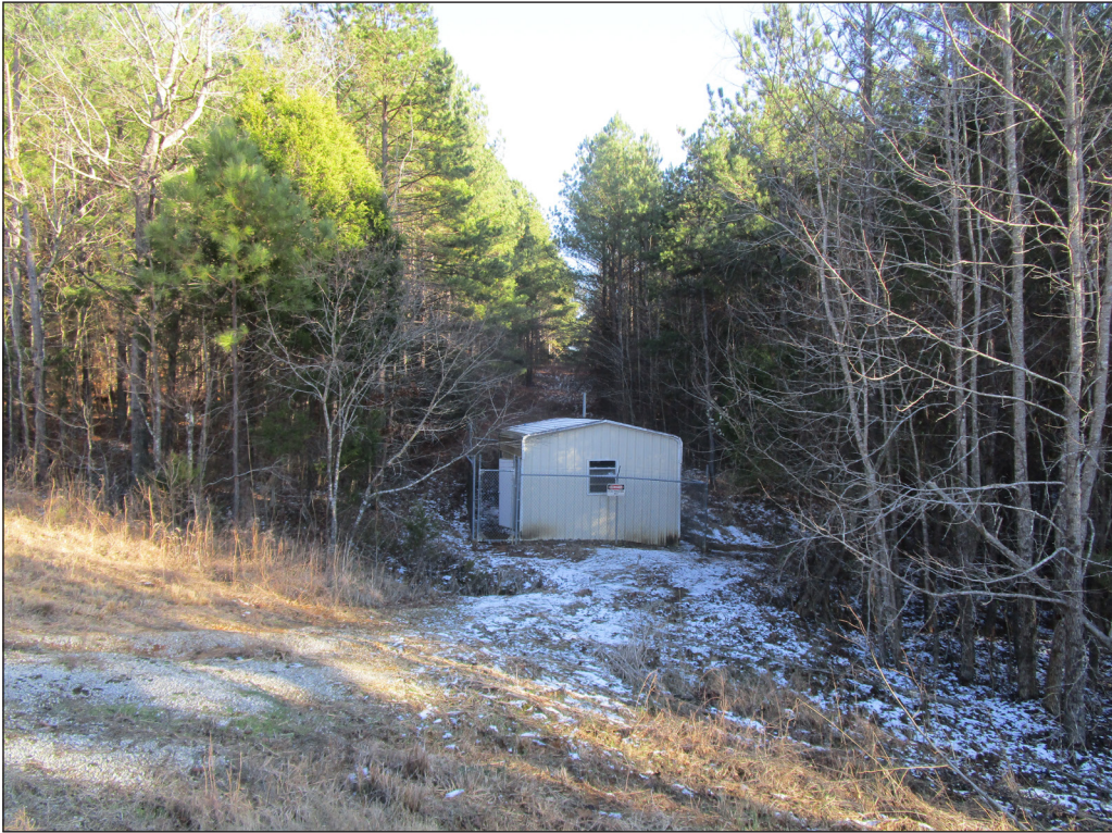
Figure 3. Western end of project route at compressor station, view southeast.
